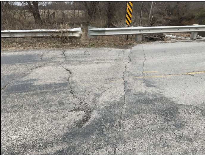
West approach roadway with asphalt settlement at the bridge end.
