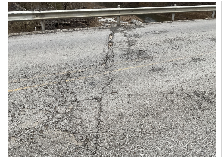
Asphalt deterioration over bent #3.
