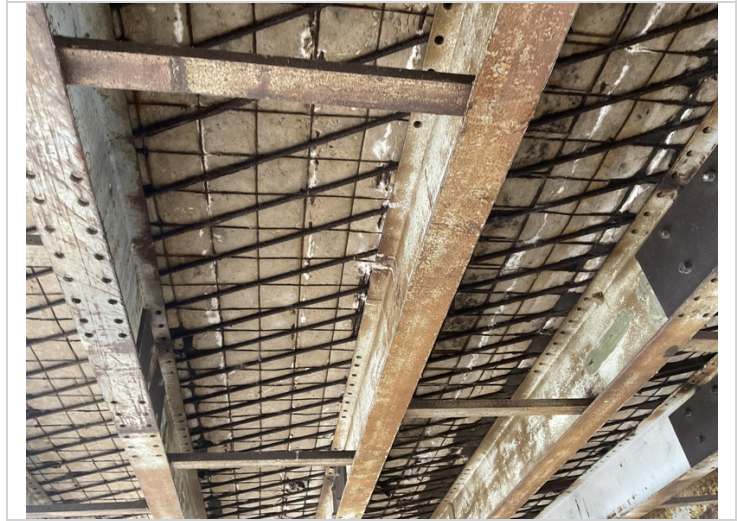
Span #3 undersurface spalling with exposed reinforcing steel.
