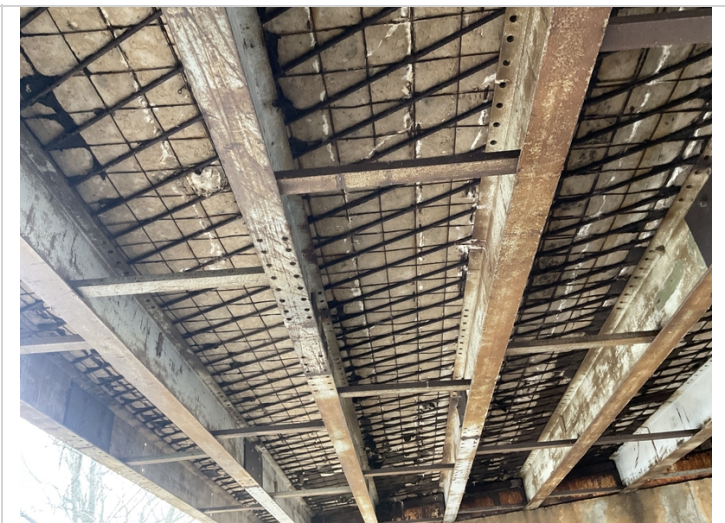
Span #3 longitudinal cracking with efflorescence buildup.
