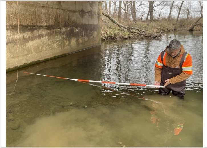
Abutment #1 footing partially undermined.
