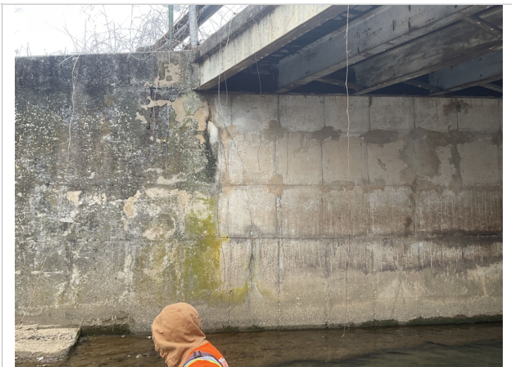
Abutment #1 Rt vertical crack at the wing wall juncture.
