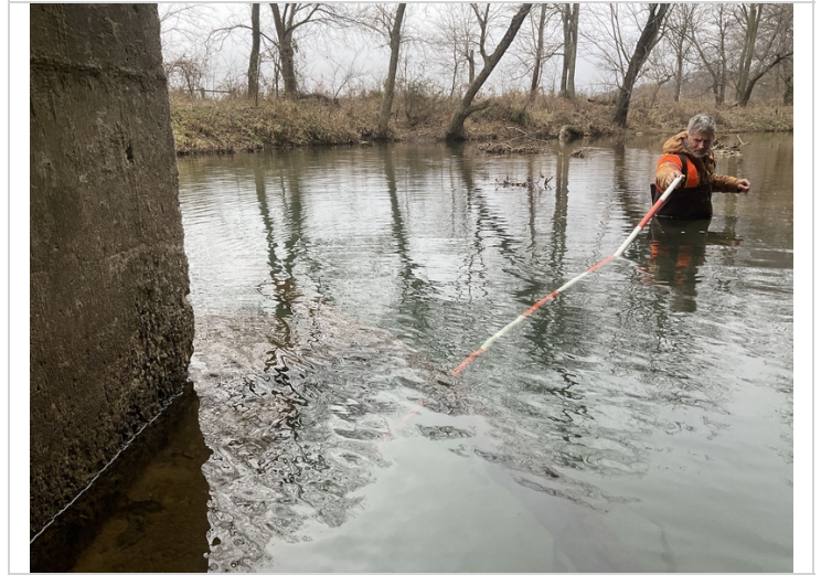
Bent # 2 inlet end with complete undermining for approximately 18" .
