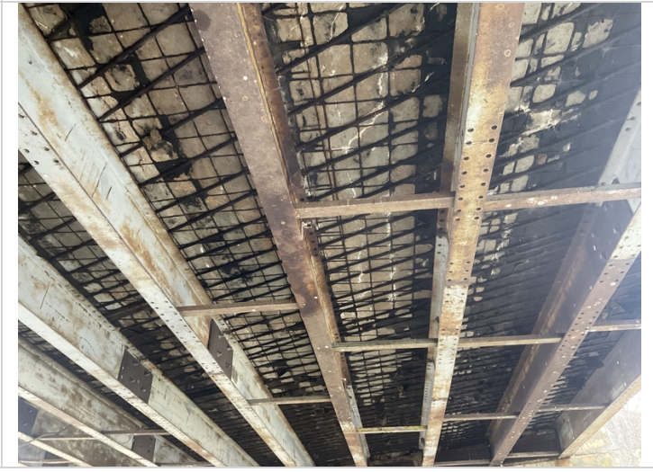
Span #1 Lt longitudinal cracks with efflorescence buildup.
