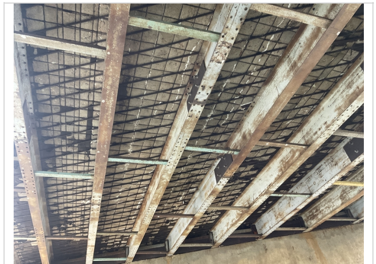
Span #2 longitudinal cracking with efflorescence buildup.
