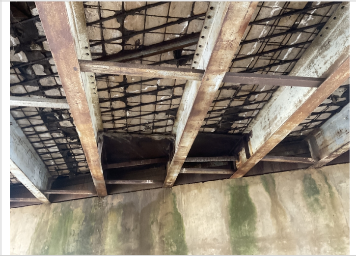
Span #3 deck repair still holding.
