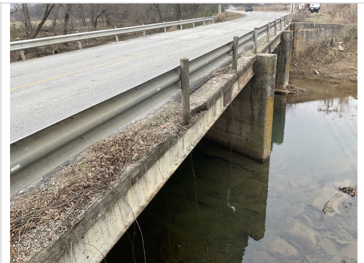
Span #1 Rt deck spalling.
