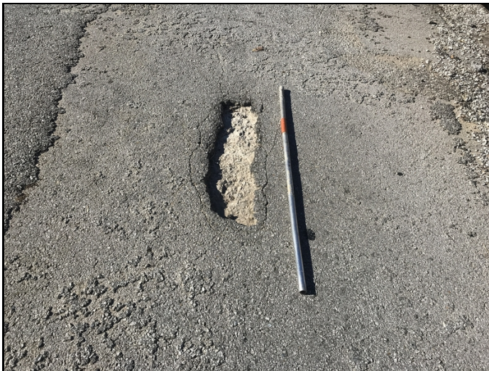
Span 2, right lane at bent # 3-Spall / pothole in driving surface.
