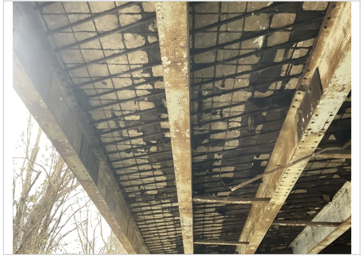
Span #1 bay # 8 & 9 spalling with exposed reinforcing steel.
