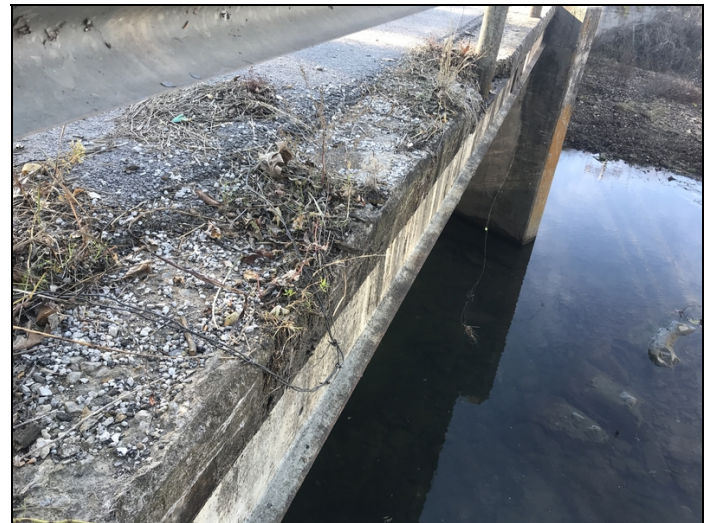
Span 1, right side-Concrete spalling / deterioration.
