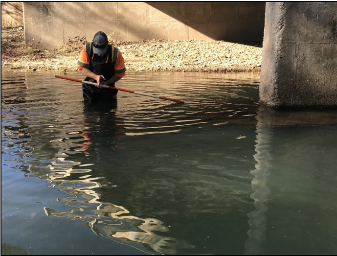
Bent # 2 left end has up to 18" of undermining. Photo # 2.
