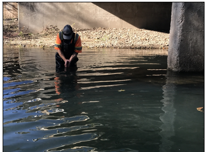
Bent # 2 left end has up to 18" of undermining. Photo # 1.
