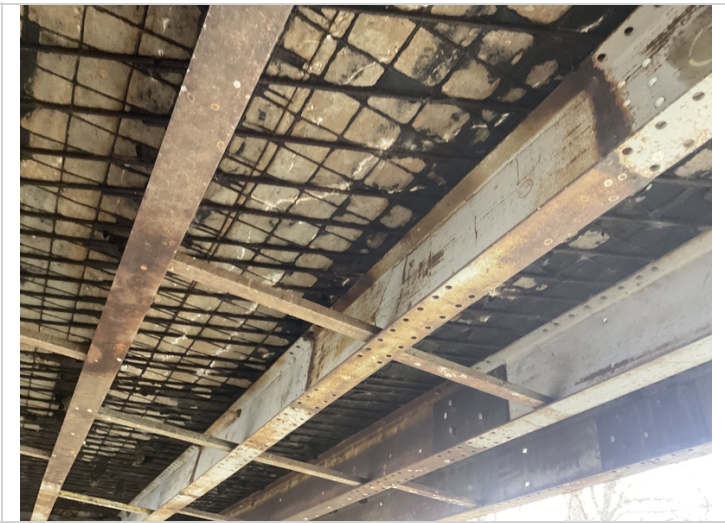
Span #1 beam #3 welded splices with no cracking visible.
